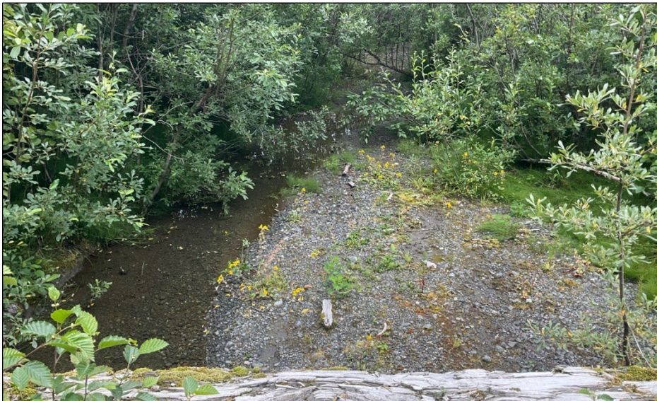
Figure 3.—Looking downstream of the bridge.
